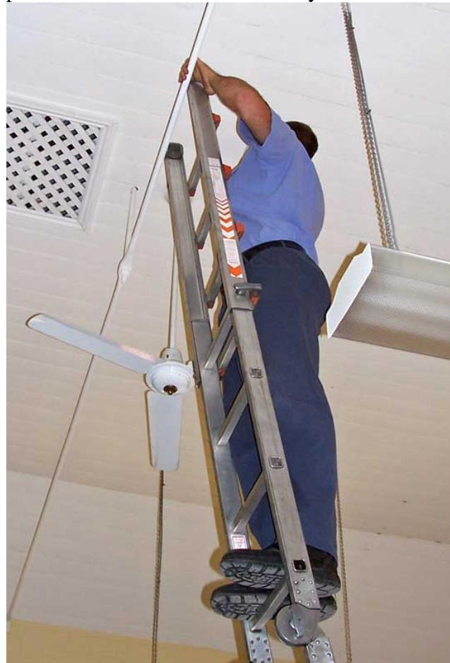
*The ladder they used is in four sections and folds up for easy carrying. They rested it on the tie rods that hold the walls together, climbed up and simply stuck the smoke alarms on the ceiling*
