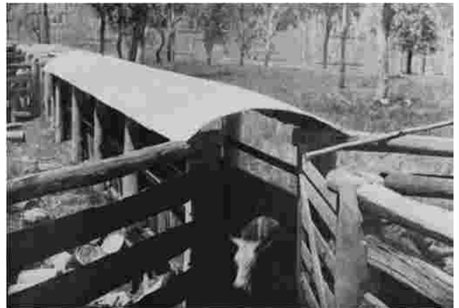
This dip was photographed at Barambah Station in 1914 and would have been similar to the Chermshire Dip which had the plunge pool covered. The gate on the exit could be swung so as to draft the cattle into either of the two yards.
