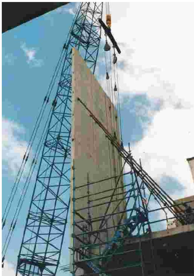
Three wall slabs being lifted into place on the south side of the Multiplex at Chermside. Very specialised equipment and a highly trained team were needed to get these concrete slabs into place in one piece. To get an idea of the size of the slabs note the worker in the bottom right corner.
