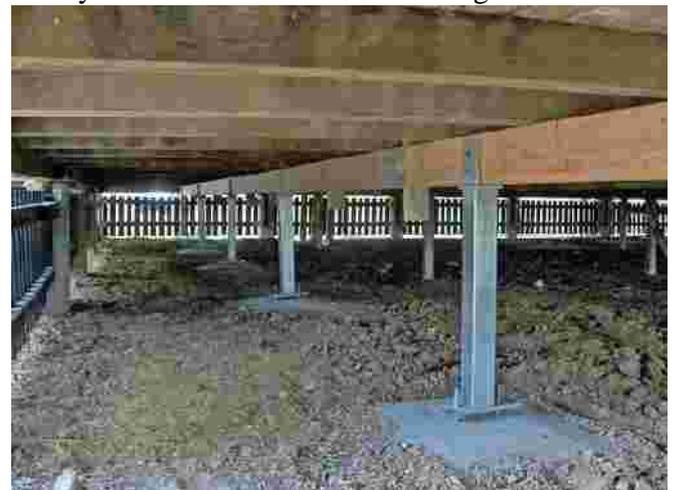
The new bearer is made of Yellow Stringybark. It is long. It is made up of two pieces of timber totaling 140mm x 75mm (5.5ins x 3ins)
