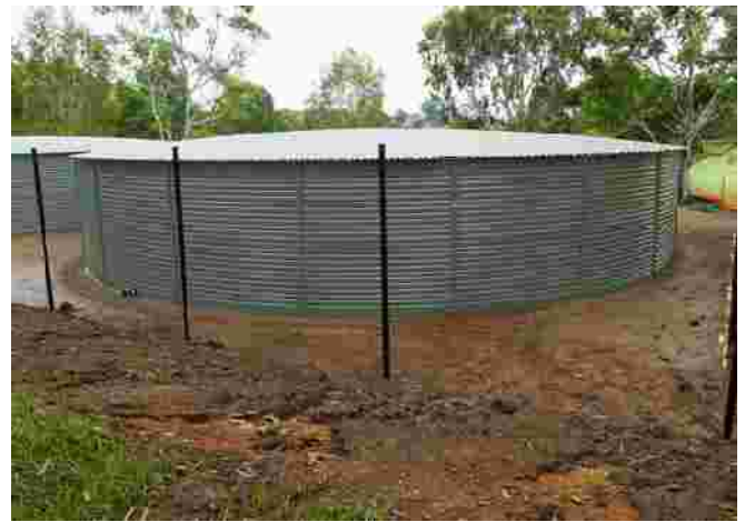
A closer view shows something of the structure.
