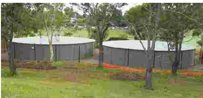
Two tanks have been erected on the above site.
