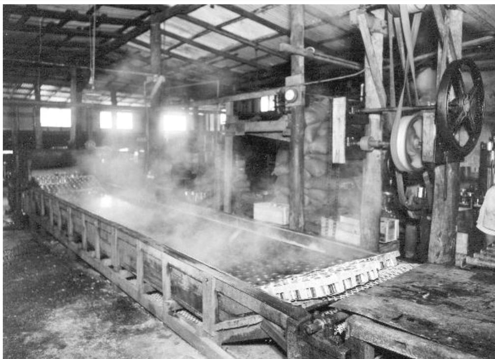
A view of the interior of Butt's Cannery in April 1956 shows the non agitating atmospheric cooker. –If any member can explain what is happening in this photo please tell us so we can classify it. Was it located in Butt Street off Murphy Road in Geebung?
